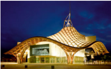
Centre Pompidou - Metz
